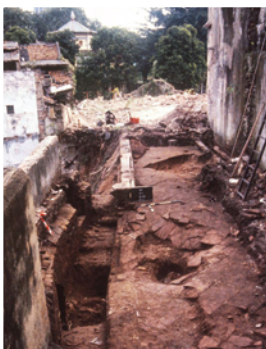
Excavations in alleyways
