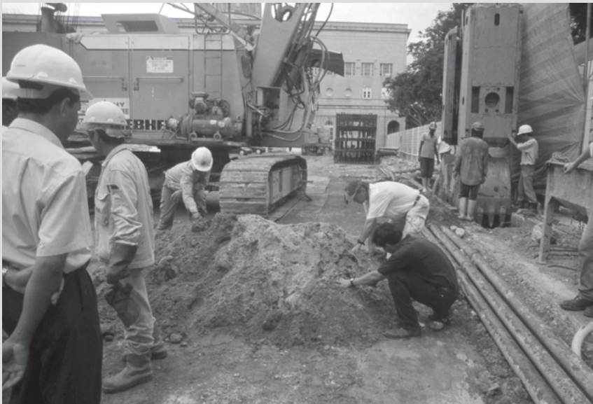
5.48, 5.49 Backhoe operations confirming the presence of fourteenth-century artifacts at CCT
