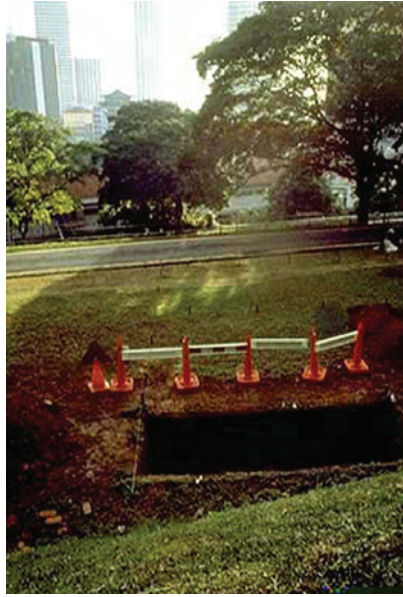
5.13 1987 ASEAN excavation, Cox Terrace
