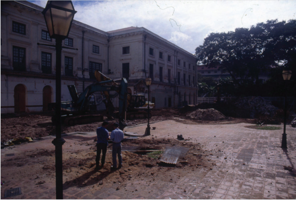
5.36 Location of first test pits, January 1998
