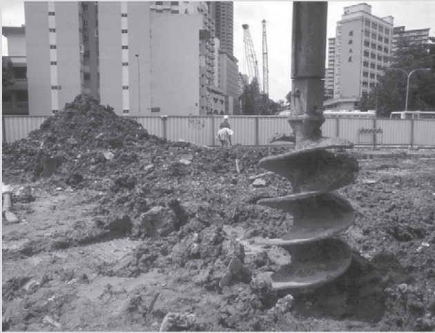
12.17 Pulau Saigon during the construction of the Central Expressway in 1990, during which the former island disappeared
