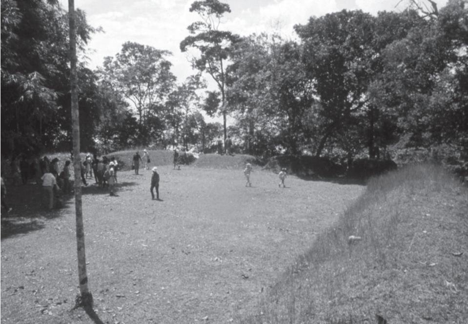
4.20 Restored bastion at the sixteenth-century fort of Johor Lama, demonstrating the use of earthen ramparts similar to the Malay Wall of fourteenth-century Singapore
