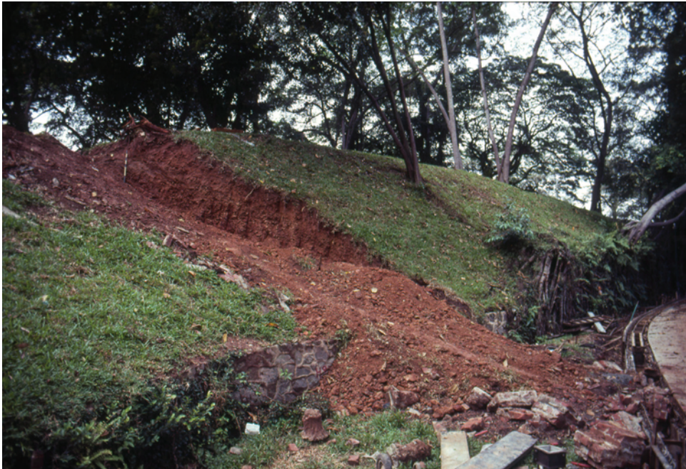
5.17 Construction of the Percival Steps revealed a layer of fourteenth-century artifacts buried beneath the nineteenth-century fortification wall of Fort Canning.
