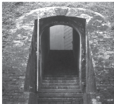
12.12 The sally port was a protected, defensive feature that allowed troops to launch attacks and retreat quickly.
