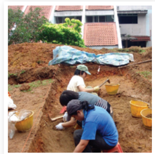
Excavation for construction of handicapped access ramp
