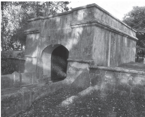
12.11 Gate of Fort Canning, built in 1860. The narrow openings at the top of the gate allowed defensive troops to fire on attacking forces.
