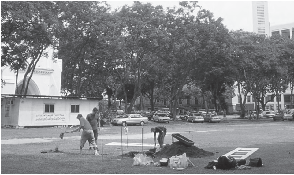
5.56 Site view, STA. Laying out the first test excavation.
